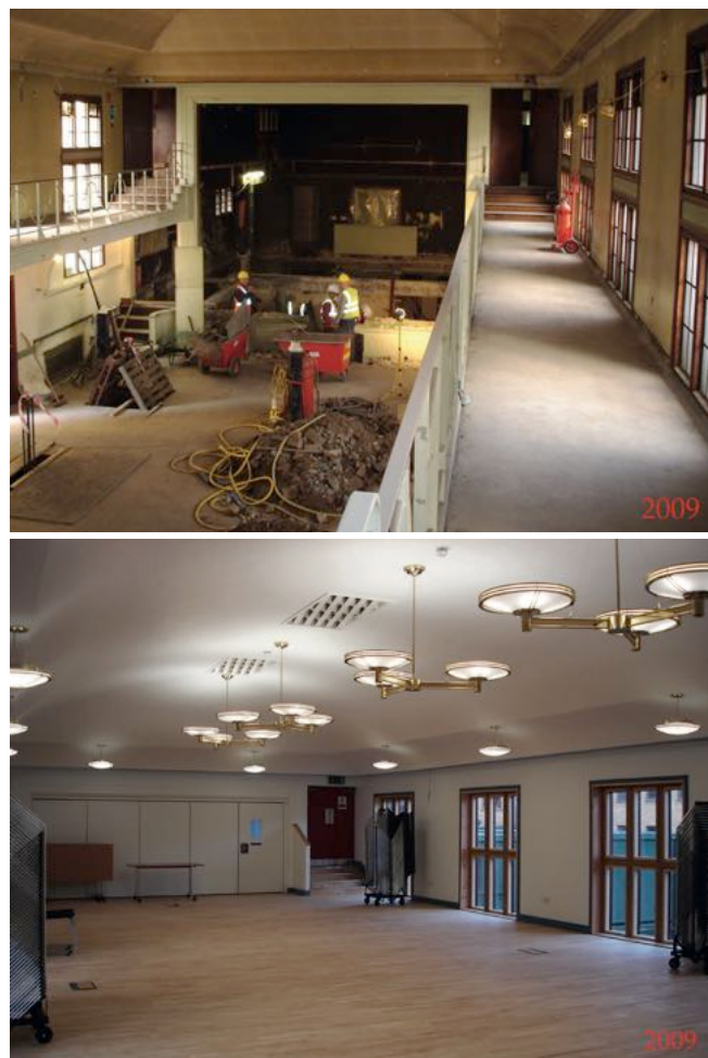
Fig. 9 View of original Hall double height theatre interior during construction and new Upper Hall on completion in 2009
