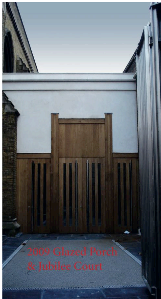
Fig. 8 View of newly installed public oak doors to glazed porch on completion in 2009
