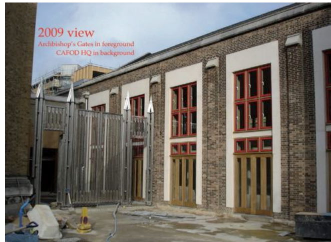
Fig. 7 View of newly ordered Hall elevations and Archbishop's gates during construction in 2009
